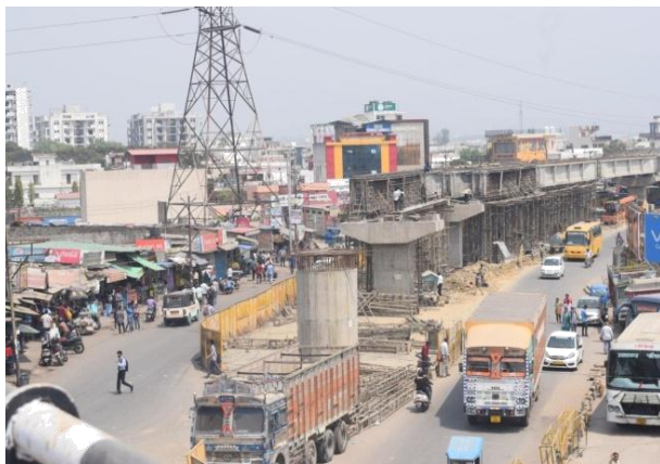
Fig 6 : View of present Dehradun (road congested)
